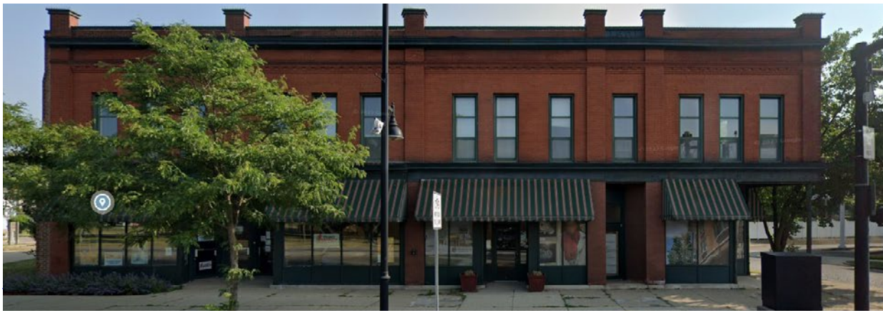
Inspiration for fabric buildings on South Main Street in Elkhart.
