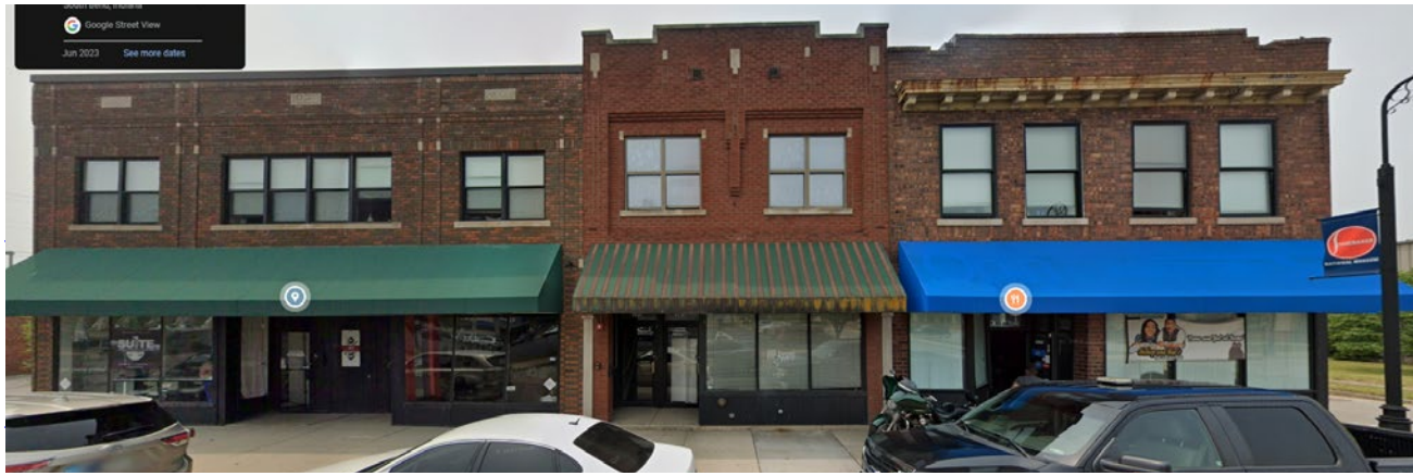
Inspiration for fabric buildings on South Main Street in Elkhart.
