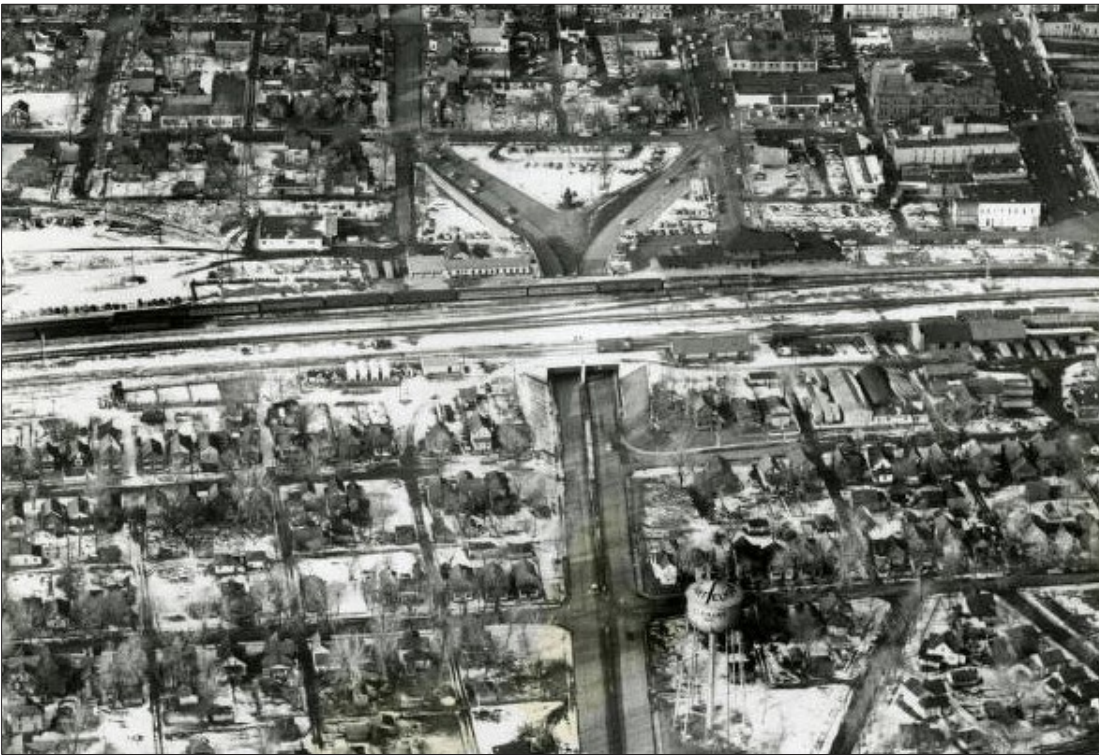
FIGURE 4: Aerial Photo Showing the Impact of the Benham Avenue Underpass, Circa 1963
